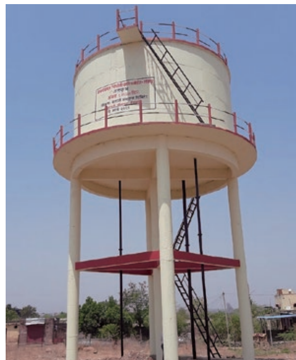
Constructed of ESR 2 Lakh capacity water tank at Grampanchayat Chincholi, Kati, Mohol, Dist - Solapur
